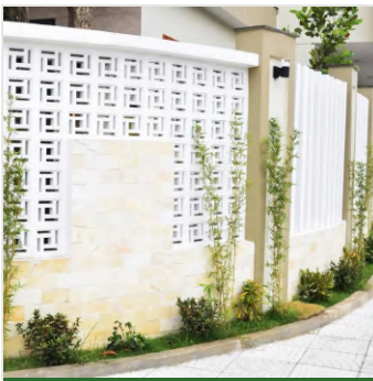
GRID Compound perimeter wall
